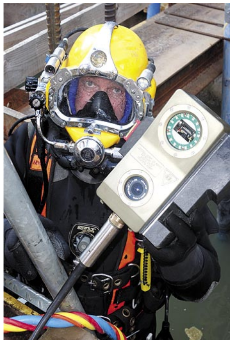
M210UW deployed by a civil engineering diver in a waterside construction site in Germany.
